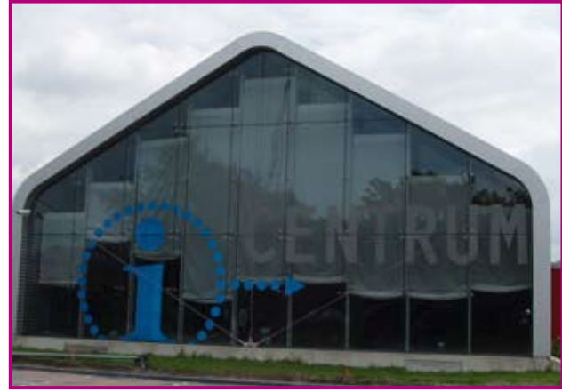
Local project team offices in new Dutch suburbs such as Vathorst improve communications
